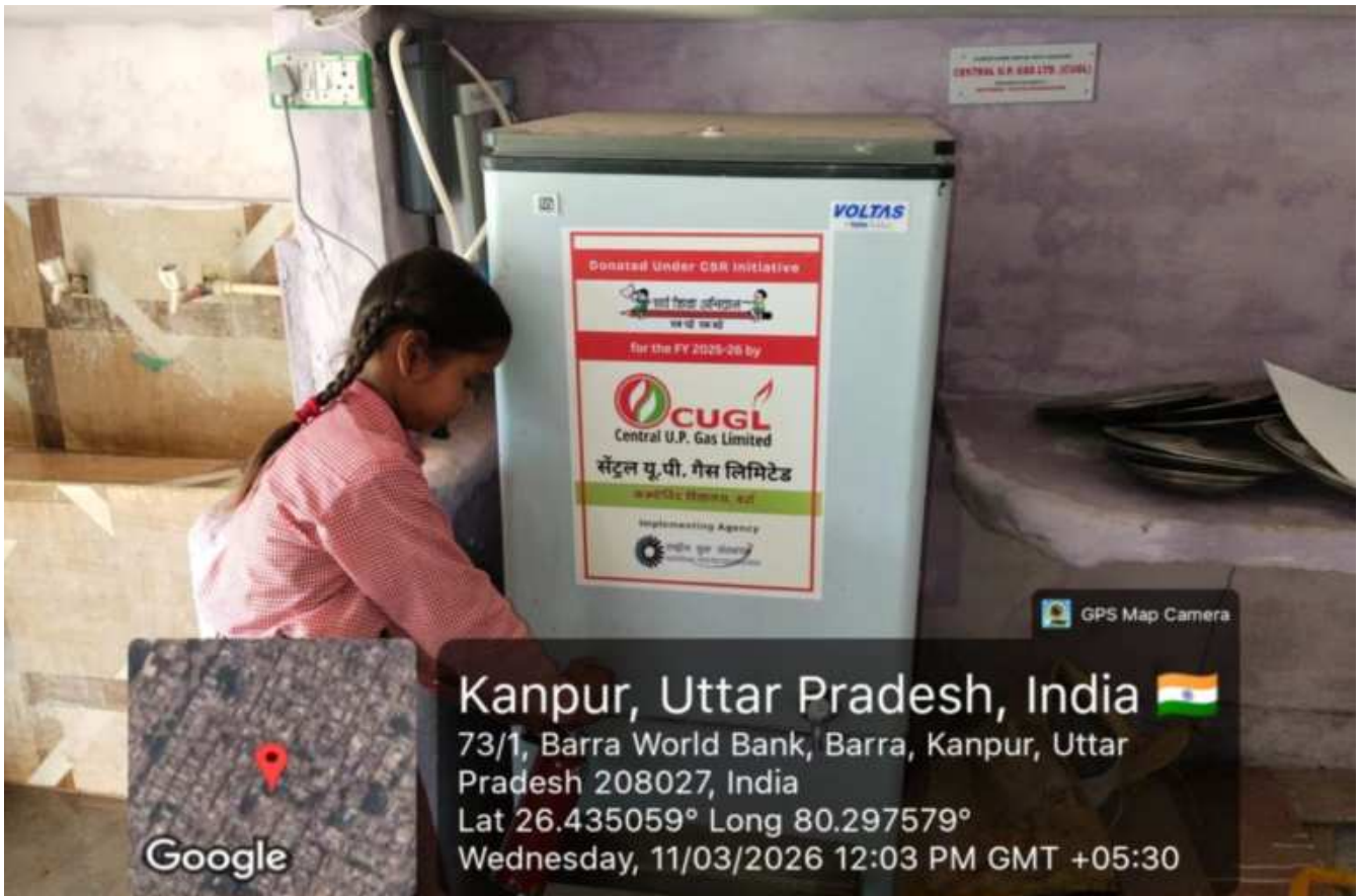
Ro & Water Cooler Installation - Government School (Kanpur & Unnao)
